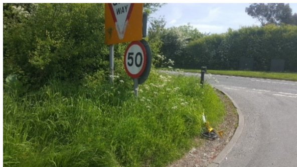
Figure 11- visibility to the left at 9m back from channel line
