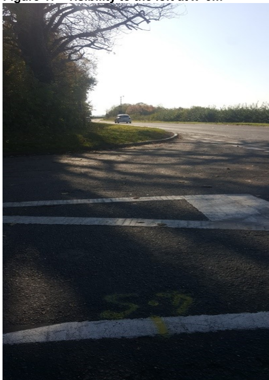
Figure 19 - visibility to the left at x=4.5m
