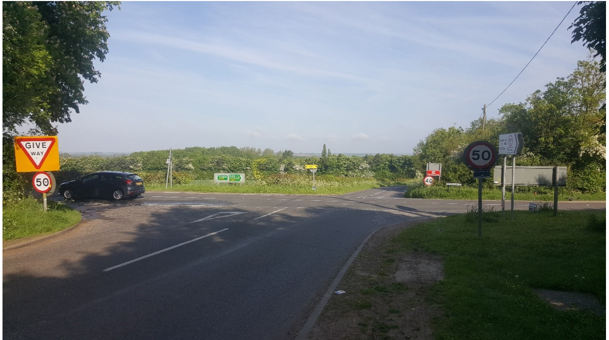
Figure 30 – view from Napton Road, confusing speed limit signing detracts from give way sign
