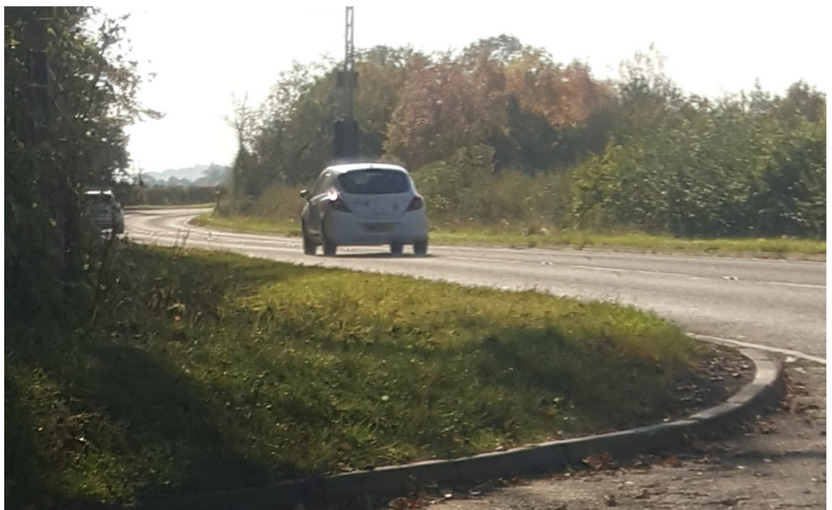
Figure 22 - visibility to the left from Napton Road at x distance of 4.5m
