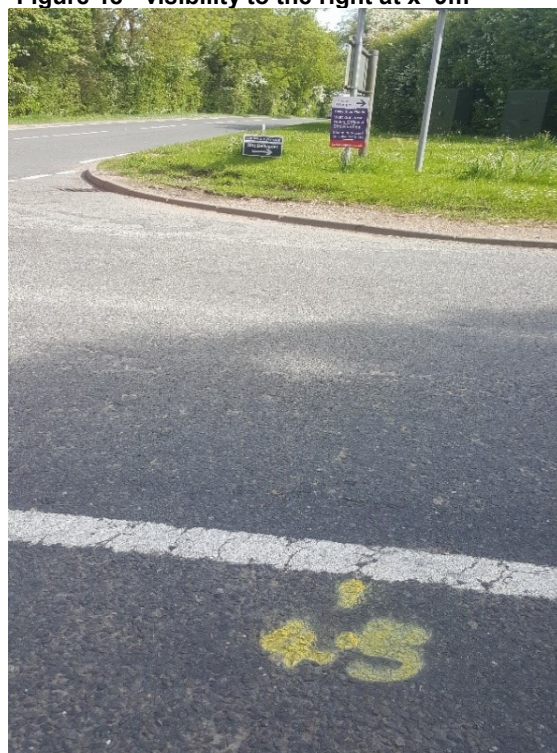
Figure 20 - visibility to the right at x=4.5m
