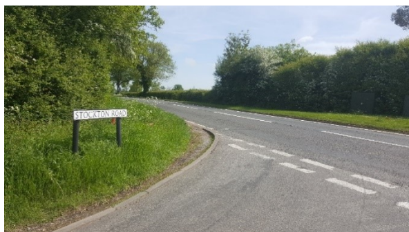
Figure 13 – visibility to the left at 4.5m back from channel line
