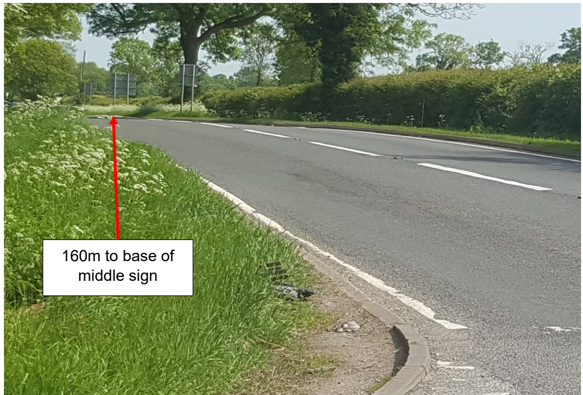
Figure 15 - looking left from Stockton Road at 2.4m x distance
