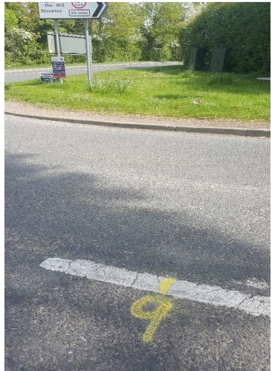
Figure 18 - visibility to the right at x=9m
