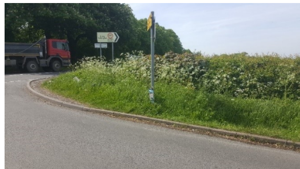
Figure 12 - visibility to the right at 9m back from channel line
